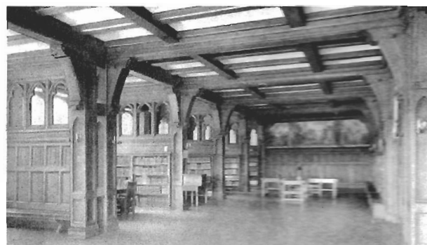
The Henry Library in 1913. The mural painted by Violet Oakley in 1905 is considered to be one of the noted artist's best works.
